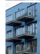
South Acton Housing Scheme
