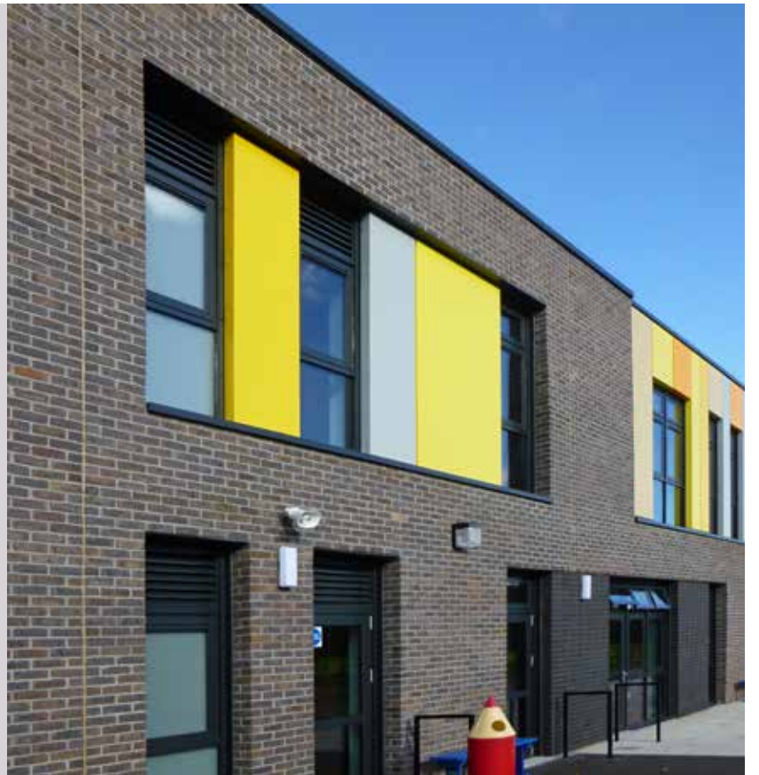
Primary School, Cambuslang, Glasgow
